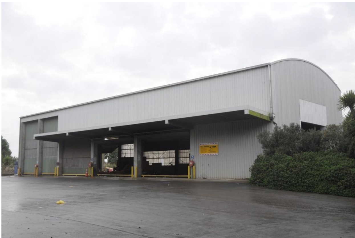
Figure 8: Invercargill Transfer Station
