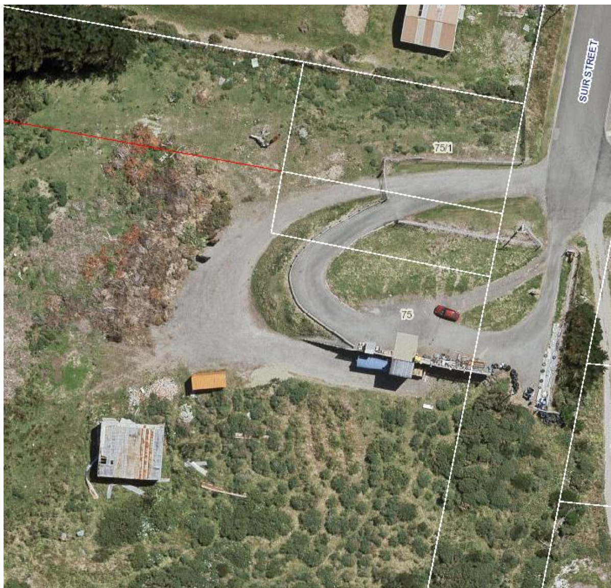
Figure 7: Bluff Transfer Station
